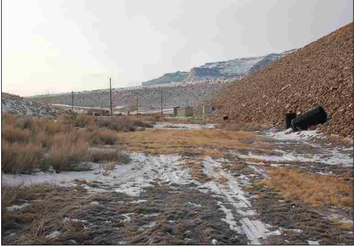
Figure 8-4. View of conditions and topography at Millsite Dam, looking south along the downstream toe of the dam, January 2015.
