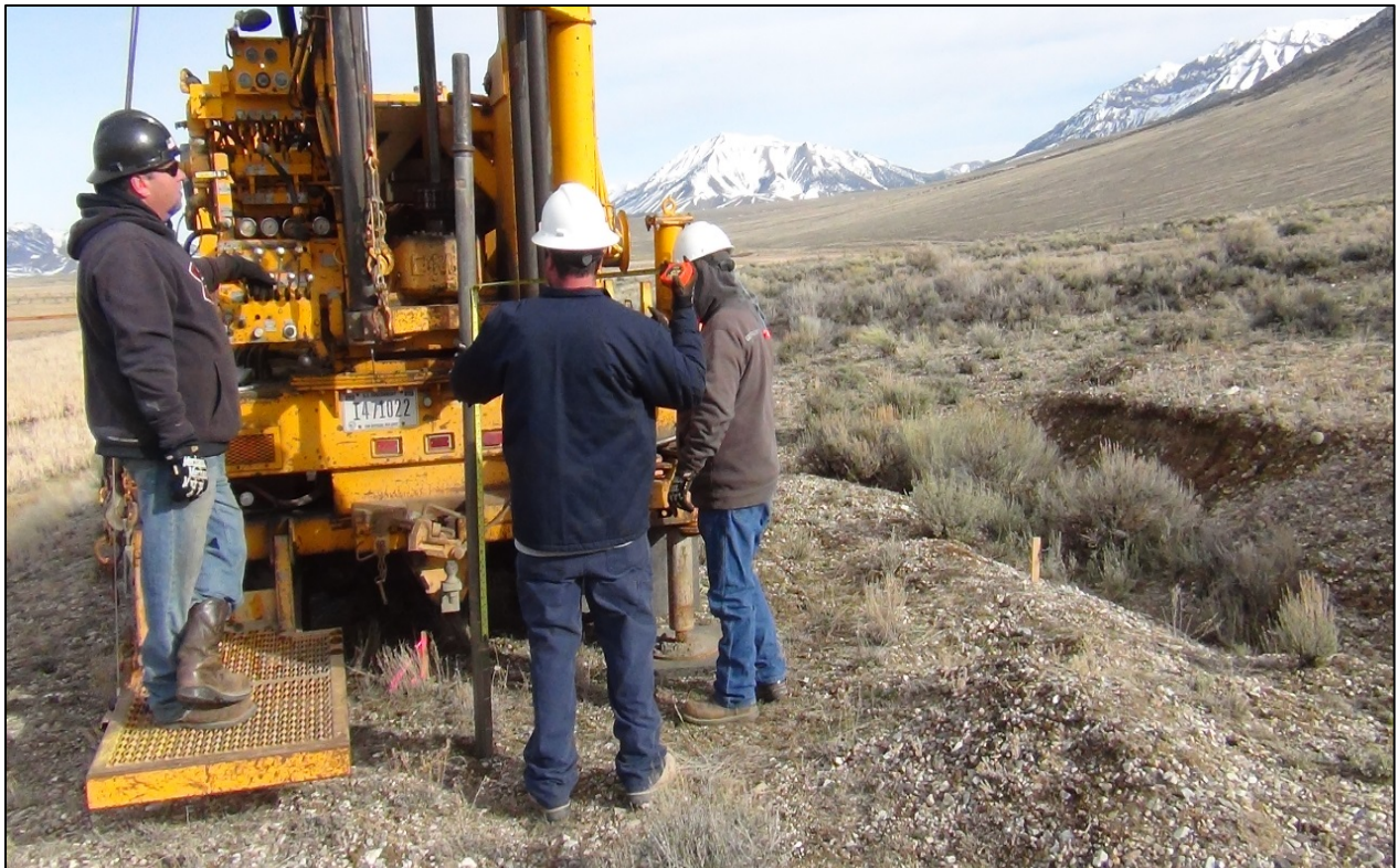
Figure 7-3. View looking north of drillers setting up on BPC-2, also showing 2017 site conditions near a large fissure caused by liquefaction induced lateral spreading towards Thousand Springs Creek to the left.
